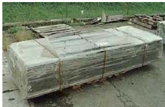
Removed asbestos sheets are wrapped with polyethylene sheeting and labelled prior to disposal
